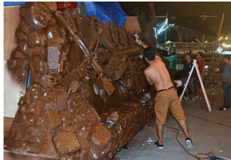
Applying the first coat of paint.
