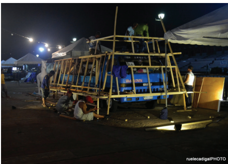
Start of the float construction.
